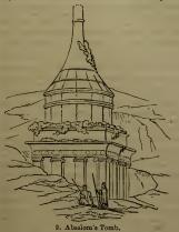
The elevation is about 18 or 20 feet to the top of the architrave, and thus far it is wholly cut from the rock. The upper part of the tomb, which is about 20 feet high (the whole has therefore an elevation of about 40 feet), has been
